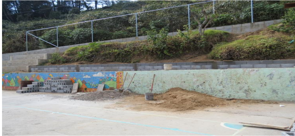
Building retaining wall above school
