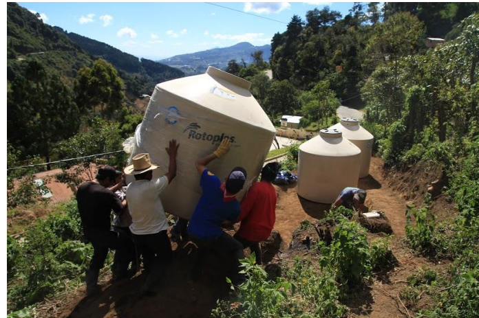
Installing water tanks
