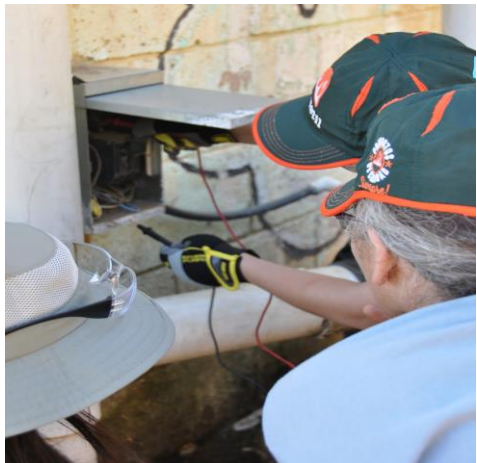
Installing water pump
