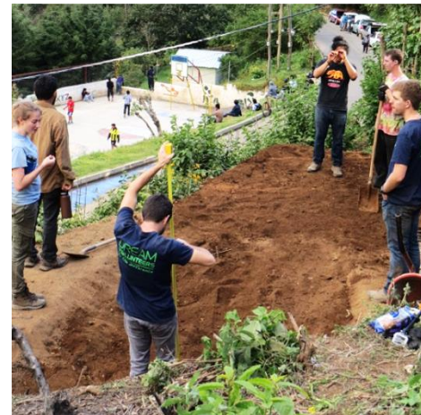
Leveling for tanks
