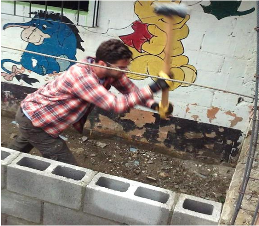
Building computer lab
