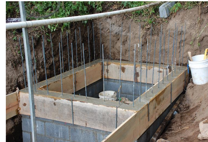
Constructing sediment basin
